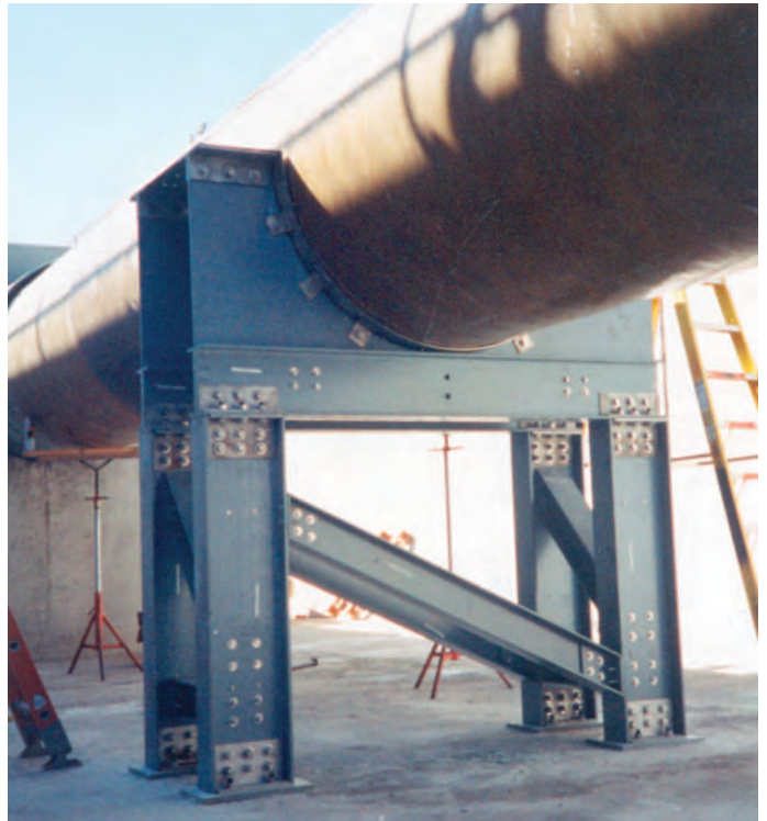
EXTREN® structural shapes were used to fabricate pipe supports to hold 1,000 lineal feet (304.8m) of 54" (1371.6mm) diameter pipe.
