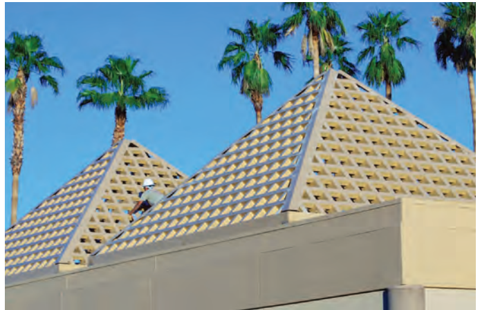
EXTREN® structural shapes were fabricated to replace the deteriorating timber pyramid screens caused by the desert's thermal cycling at the Vintage Club in Indian Wells, California.
