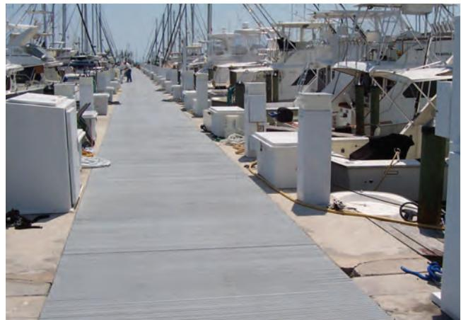
Strongwell's DURAGRID® T-1700 pultruded grating was used to replace wood planks on a large walkway at Dinner Key Marina in Miami, Florida. The grating allows for easy accessibility to utilities below the walkway and will not rot like the previous wooden walkway.
